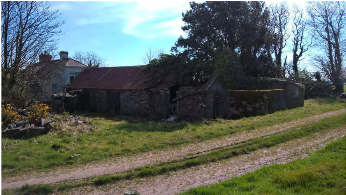
Photo 1: View of extant 19 th century farm buildings (58-61) within the site boundary in the southern half of Ballydaniel townland, west of Park Hill Road, looking south-east.
